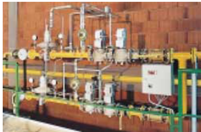
A correctly sized fuel train provides even flow of fuel to the combustion system throughout the operating range of the system.
