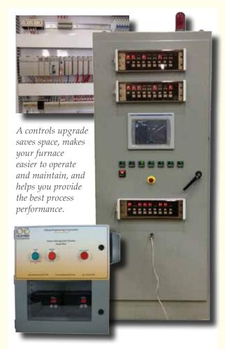
Olsträd upgraded a 24-burner reheat furnace, replacing the Honeywell flame safety panel with space-efficient Kromschröder PF-19 burner controls. An Allen-Bradley CompactLogix controls and supervises the furnace and thermal oxidizer.
